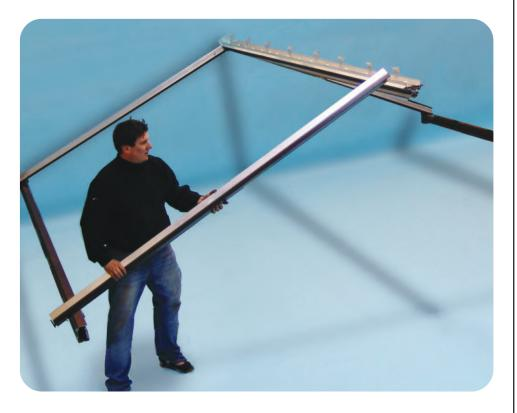
Now working from left to right viewed from outside, fit all the side transoms, by locating the pins into the ring beams, then then aligning the transoms with the holes at the top with those pre-drilled on the ridge. Now fix at top and bottom using the short wide self tapping screws provided.
