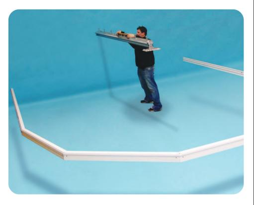
Support the ridge with a suitable prop, ensuring that the ridge is level.
