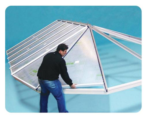
Glaze the front of the roof starting with the left hand side and working anti-clockwise viewed from outside.
