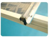
Check that the aluminium foil to the top and sides of each panel are undamaged. Now working anti clockwise, viewed from outside select roof sheet 1, peel back the protective film on each side of the panel so that the roof can be glazed.
