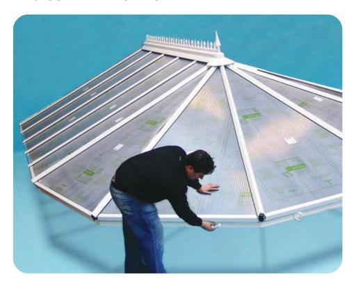
If not pre-fitted please ensure the external ring beam fascia is fitted to the mill finish ring beams.
